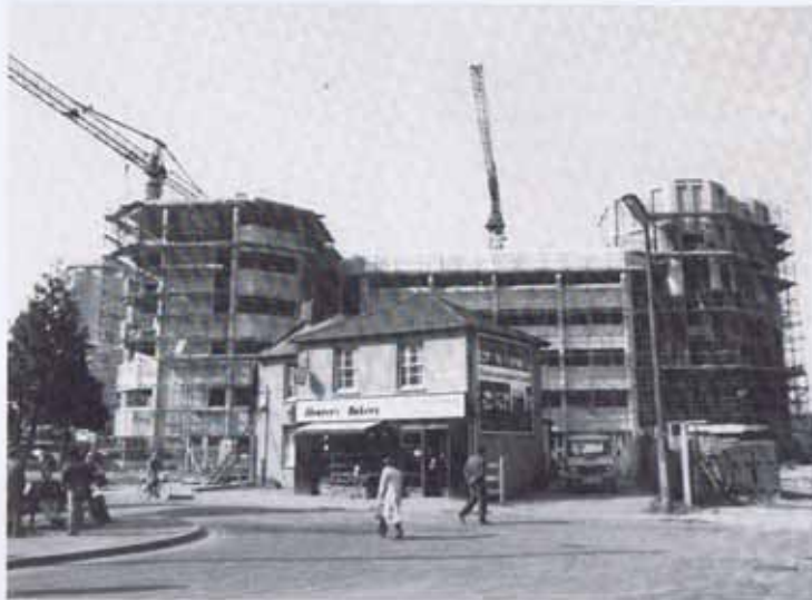
Woking Council Offices, as seen from Chobham Road, under construction in 1983
