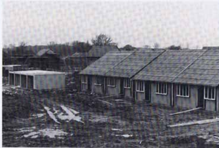
Part of Goldsworth Park under construction – c. 1980
