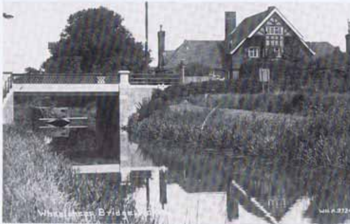
Wheatshaf bridge after being rebuilt in 1913-14.
