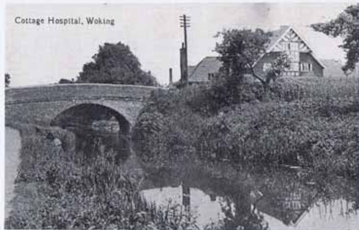
Wheatshaf bridge before reconstruction
