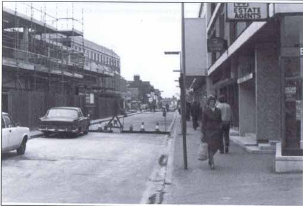
The new town centre under construction along Commercial Road – later renamed Commercial Way.
