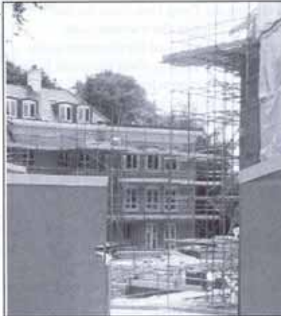
Above - Construction of the crescent at 'Brackenbrae' off Heathside Crescent.
