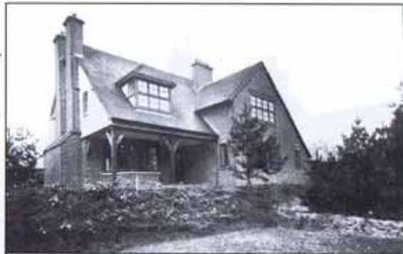
Ganges Lodge in Pembroke Road, designed by C.B. Tubbs and A.A. Meser and built in the early 20th century by Messrs. Drowley & Co. of Bath Road, Woking.
