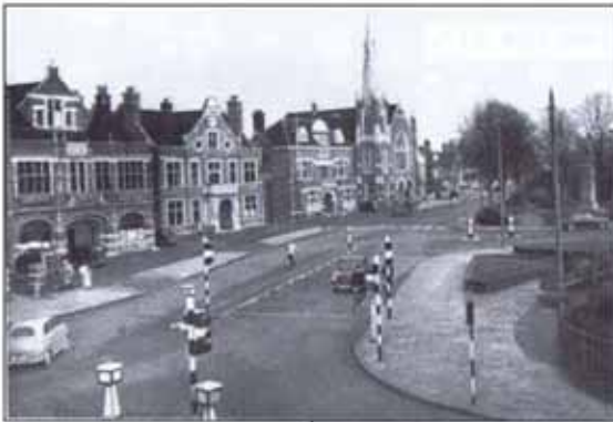
Above – The public buildings again showing the mass of traffic lights that were eventually installed to control the junction of Commercial Road, High Street, Goldsworth Road and Percy Street by Victoria Arch.
