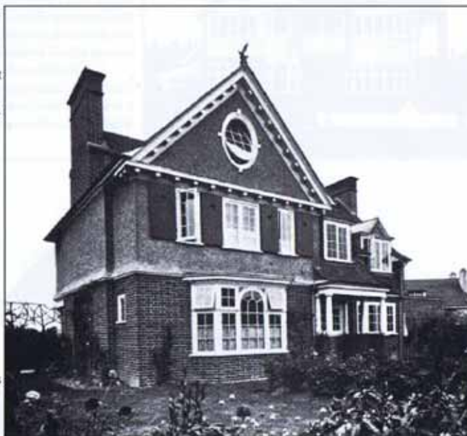
Normanhurst in Heathside Park Road was another property built by Drowley and Co. in the early 20th century. In their brochure of 1907 it is described as "built of red bricks, with orange rough cast, dark tiles, and green shutters".
