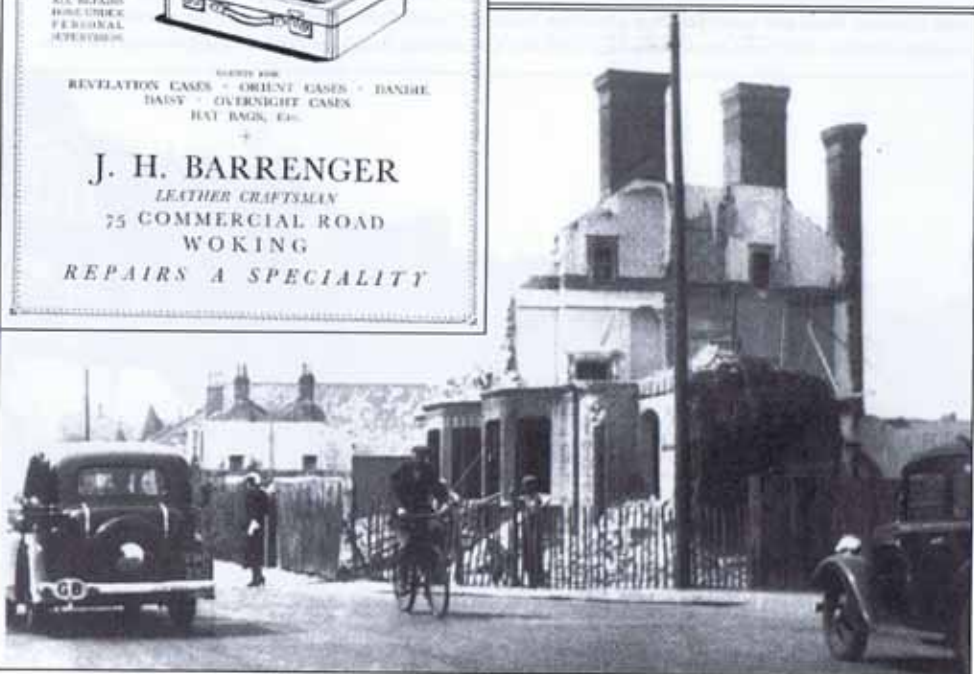
Below - The houses of Commercial Road, between Church Path and the Atalanta Ballroom, on the corner with Bath Road, were demolished in the late 1930s. When the car came the land was used as a car park until the mid-1970s when the new town centre (Wolsey Place) was built on the site.
