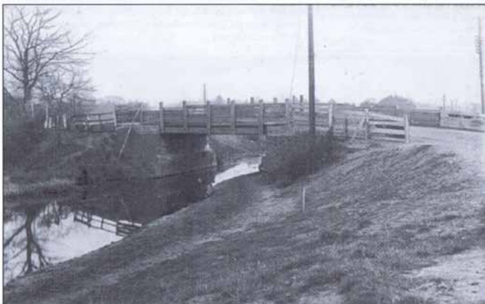
The old brick arch bridge at Chertsey Road was so bad in the early part of the 20th century that in the autumn of 1906 it had to be closed. The Council then replaced it with the 'temporary' wooden bridge (above), before finally replacing it with the current bridge in 1922.
