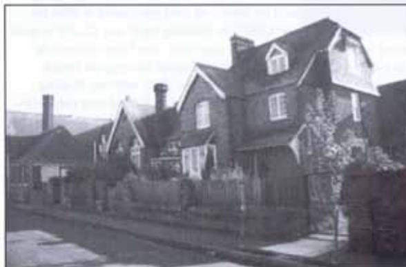
The headmaster's house in Board School Road.
